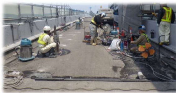
床版吊り孔削孔
