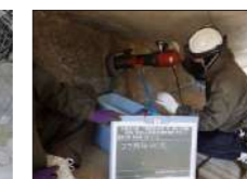
中能登土木橋梁補修
