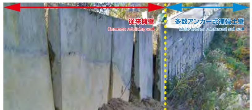
被害が発生した従来擁壁(左手前)と、持ちこたえた多数アンカー式補強土壁(右奥)。Common retaining wall that suffered damage (left side, toward the front), and a multi-anchor reinforced soil wall that held up (right side, toward the rear).
